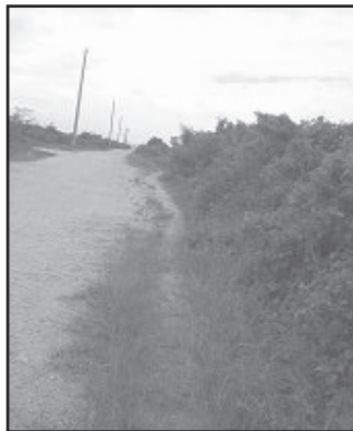
Bringing electricity to Casa de Luz: electrical poles erected this month
